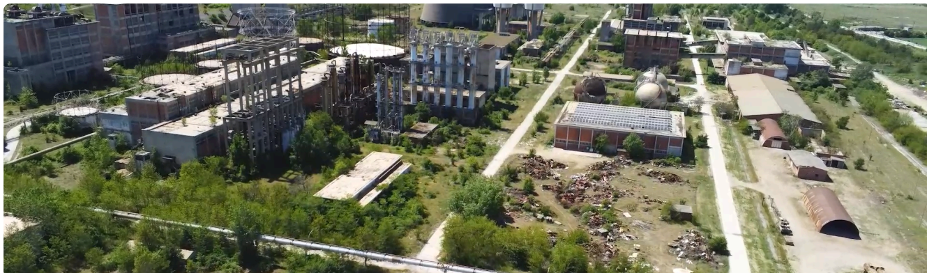
The former AEVAL industrial site in Ptolemaida, Western Macedonia — 506,000 m 2 slated for demolition and environmental rehabilitation.
