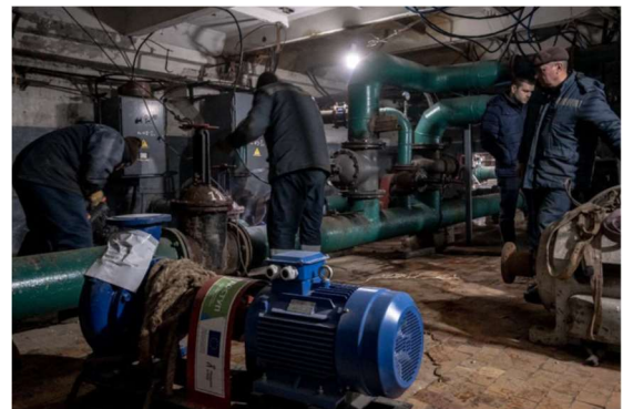
PIN Water Supply System Support in Ukraine (2024)
