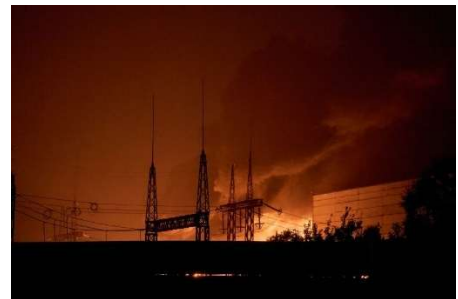
The thermal power plant following a series of explosions in Kyiv, Ukraine, October 2025 (CNN)
