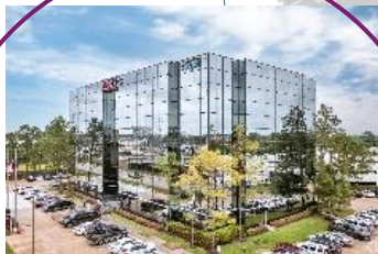
Bioprocess Center (C4B) Houston, Texas, USA (2023)
