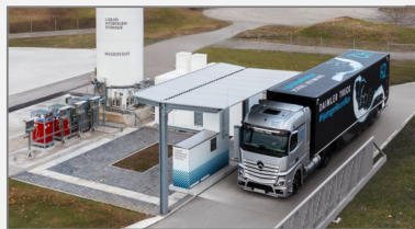
Hydrogen refilling stations for HDT (700bar/sLH; > 50 kg H 2 /single fill)
