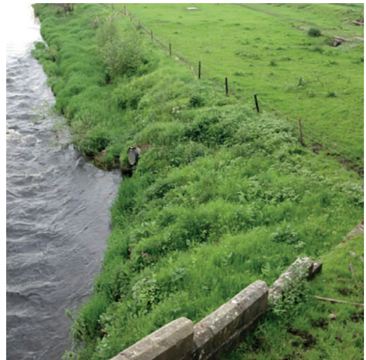
Loyn Bridge 2024, Lancashire
