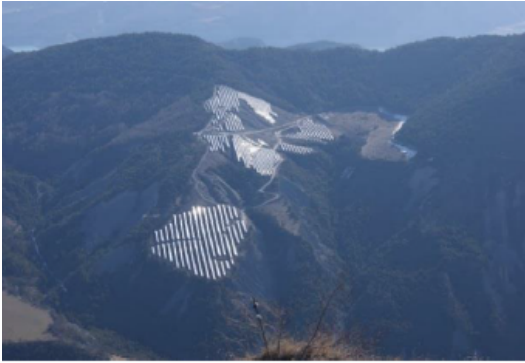
Espinasses solar field France
