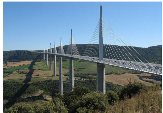
Millau Viaduct France
