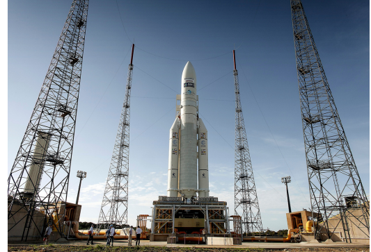
Kourou Launching Station Guyana
