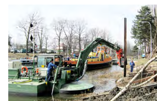
Strengthening shorelines by pile driving
