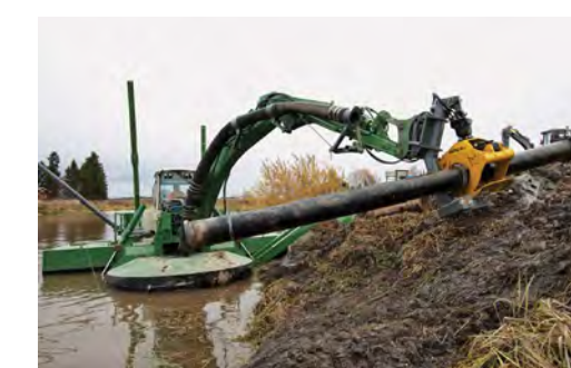
Trench digging and laying underwater pipes and cables
