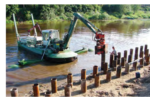
Foundation work by pile driving
