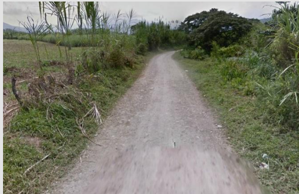
Current status of the road San Gil - Mogotes
