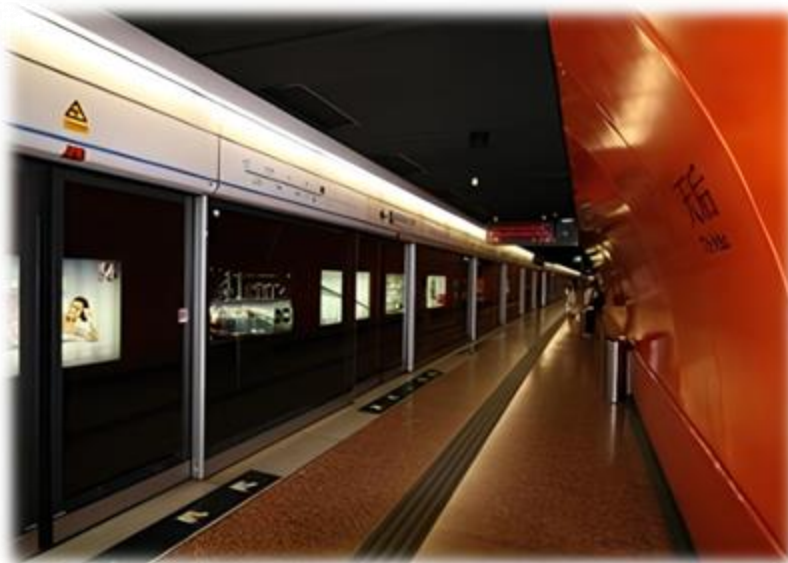
Platform Screen Doors (MTRC) (150 platforms)
