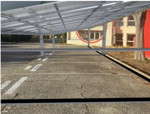
(June 2025) Low- carbon solar PV carport 100 sqm / 25 kW
