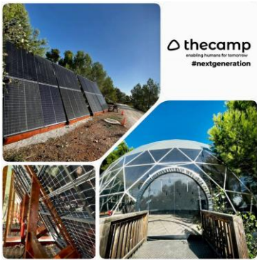
(2022) Zero-carbon solar PV power plant 42 sqm / 17.5 kW
