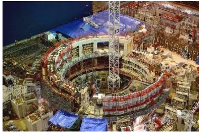
Architect-Engineering and Construction Management for all buildings and auxiliary systems at ITER Site
