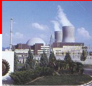
Trillo NPP, Spain PWR, 1066 MWe Framatone (Siemens-KWU)
