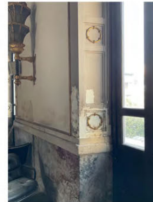
test on paint and plaster
