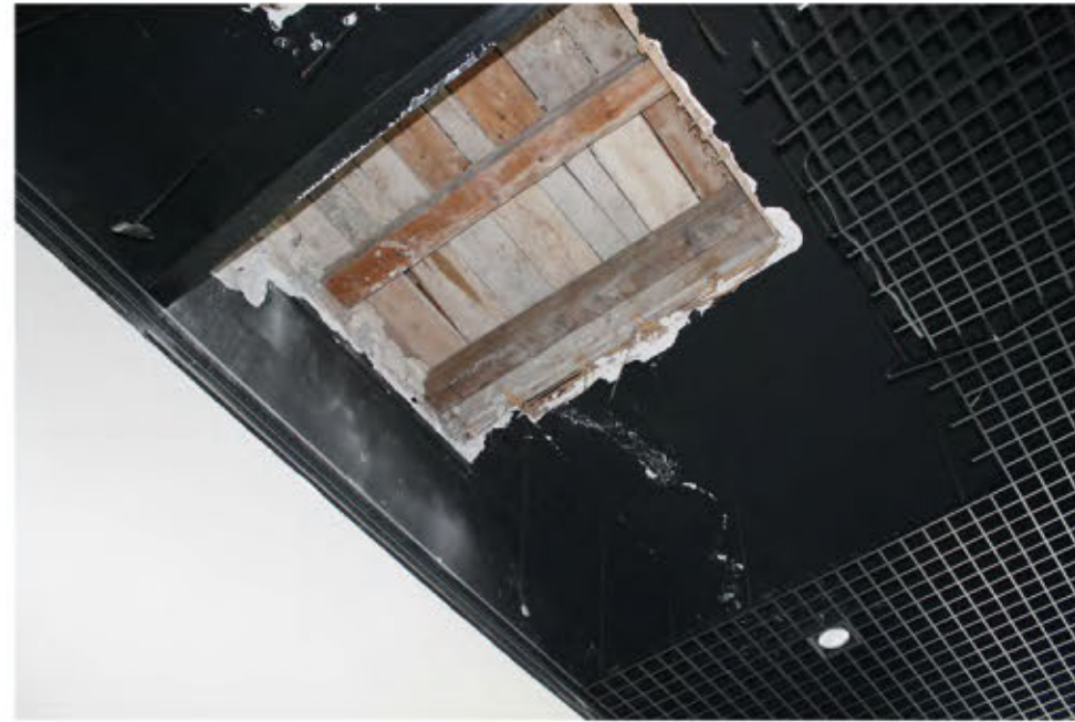
structural test on slab
