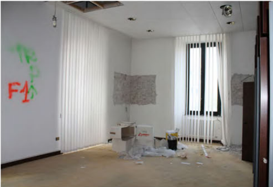
structural test on wall
