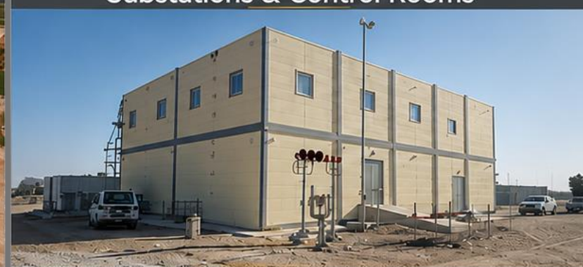
Prefabricated E-House / Substations & Control Rooms
