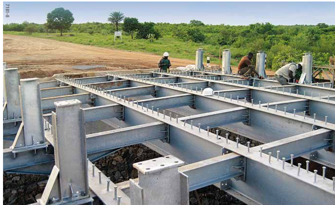
Far Left: Continuous composite beam bridge, Maphutsaneng Bridge, on the Mophale Hoek-Mekaling road, Lesotho - Africa.
