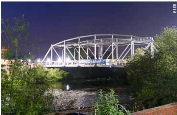
Above: Lifting a 46m span bridge into position in Rotherham, UK. Right The same bridge in position.
