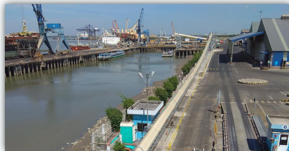
Tubular Belt Conveyor
