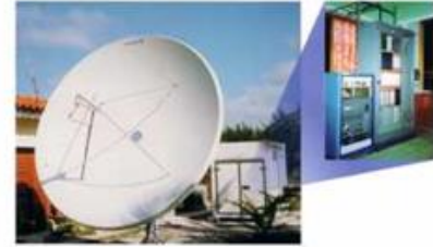
VSAT Rural Network Remote sites with Ericsson Edge Small Public Exchange
