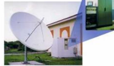
VSAT Rural Network Remote sites with Ericsson Edge Small Public Exchange
