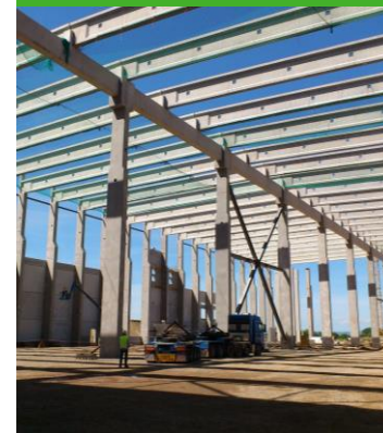
Prefab. industrial (pillars, beams)
