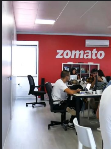
Zomato - Portugal HQ Office renovation
