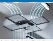
Passive cooling takes advantage of the naturally occurring temperature swing caused by day & night. The excess coolth available in the night can be stored in the PCM, which is then released during the day absorbing internal and solar heat sains.
