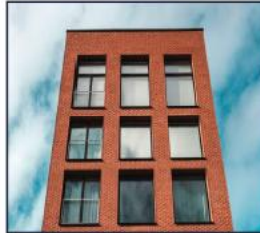
CHP for Buildings
