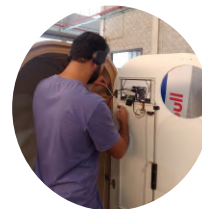
Maintenance and technical support
