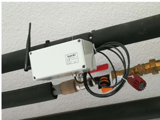
↑ ISURLOG-LR field unit measuring diverted water temperature and flow.
