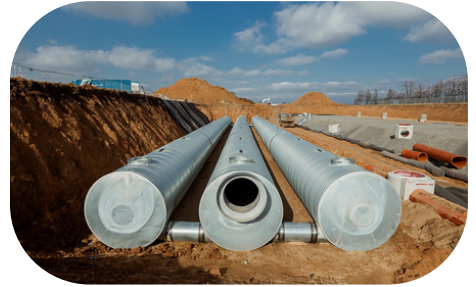
Stormwater solution for NEXEN Tire plant in Žatec, Czech Republic 1,200m 3 of corrugated steel pipes
