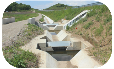
Stormwater treatment at the Lugoj-Deva highway, Romania ENVIATRP oilseparators were installed
