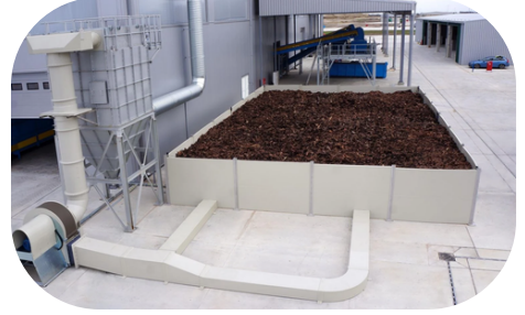
Air treatment project at a waste management centre, Subotica, Serbia Capacity: 20,000 m 3 /h
