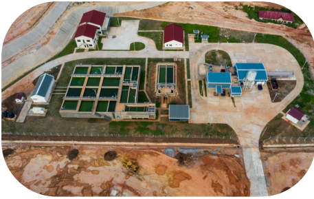
Faecal Sludge Treatment Plant in Kumasi, Ghana Capacity: 1,000m 3 /d Budget: 10€ million
