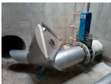
VORTEX installation after a infiltration / detention tank.
