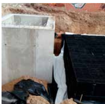
VORTEX installation after a infiltration / detention tank.
