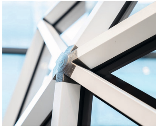
VISS 3 3D printed steel nodes
