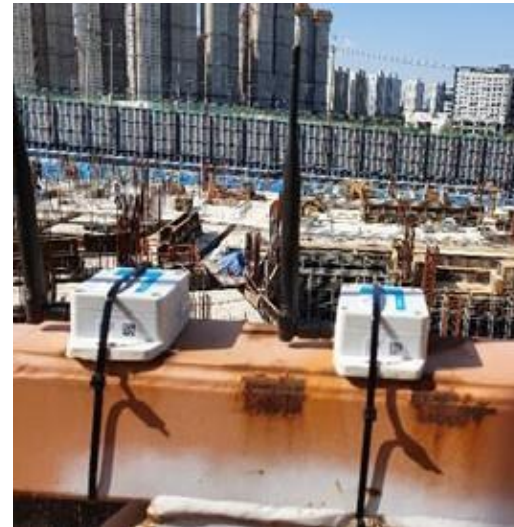
Hanhwa Construction (2020.04) Comprehensive monitoring of the construction site
