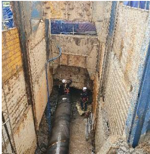
SK Construction (2020.11) Collapse prevention of support structures
