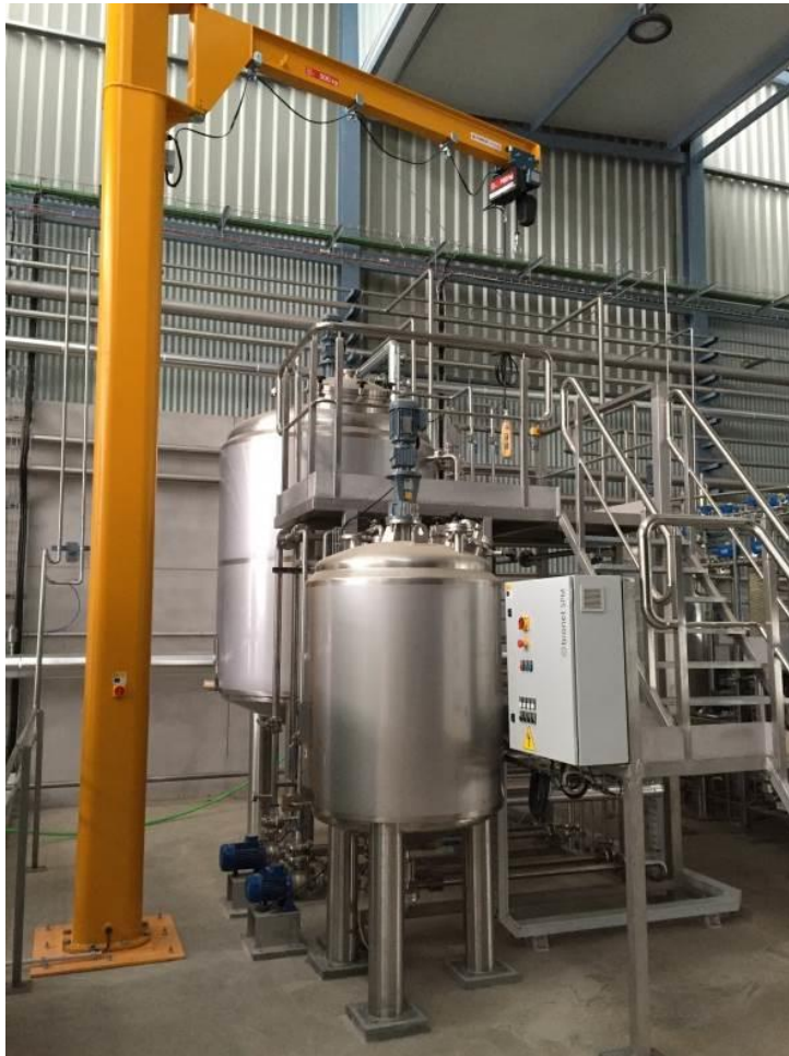
Substrate preparation system
