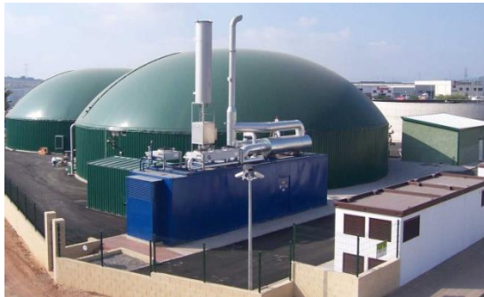
Anaerobic Digestion
