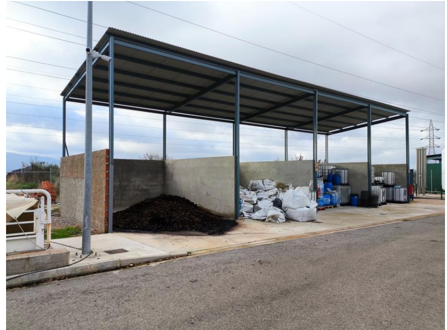
Solid biomass storage silos
