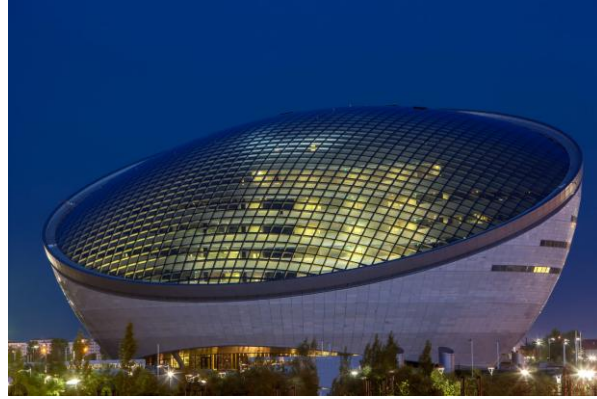
Façade & Roof Cladding
