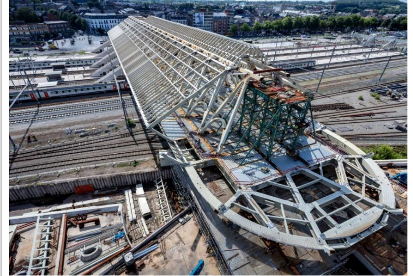
Heavy Lifting & ILM Works
