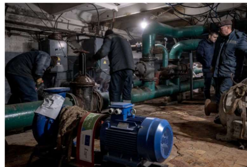
PIN Water Supply System Support in Ukraine (2024)
