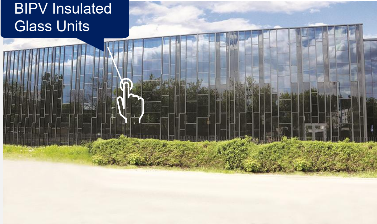
Project completed in 2021 for Medical University in Warsaw, Poland, 720m 2 BIPV Insulated Glass Units (IGU) in Curtain Wall
