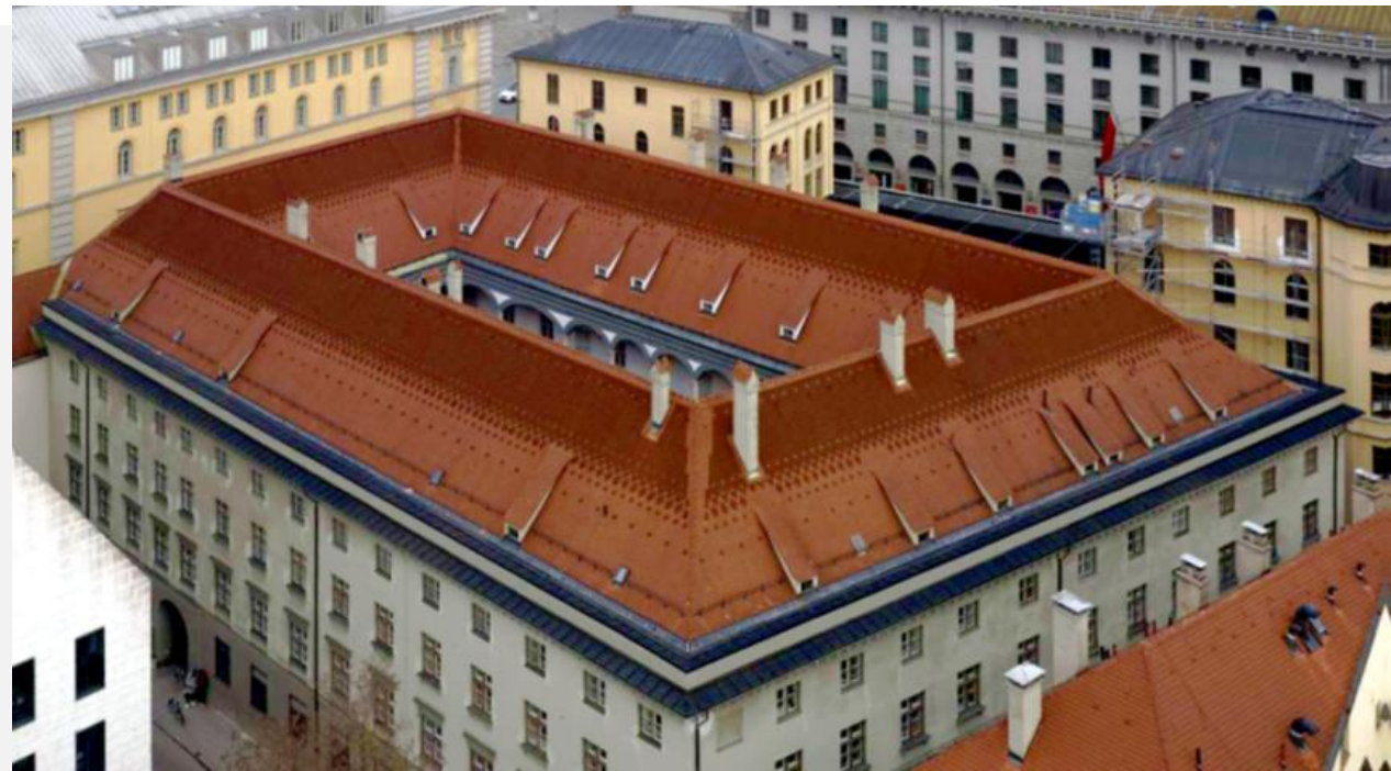
Ongoing project for renovation of XVI century historical building in Munich, Germany. 400 sqm PhotonRoof, Carptiles Red. Headquarters of the Bavarian State Office for the Preservation of Historical Monuments.
