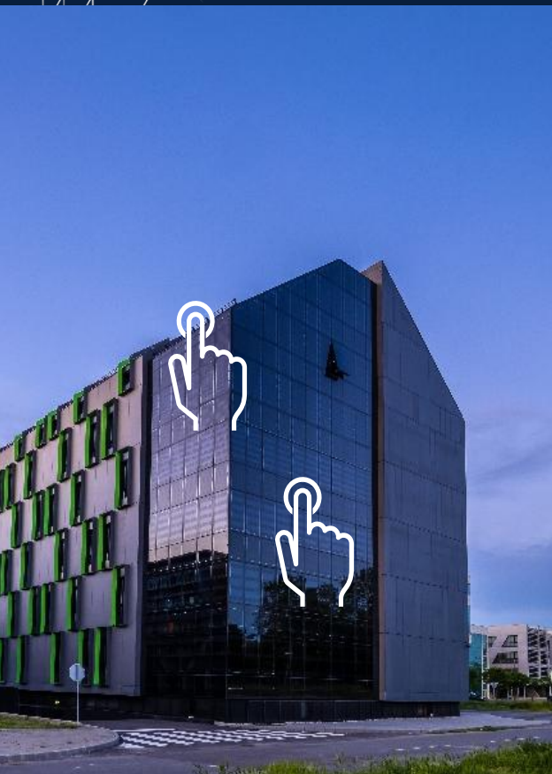
ML System supplied transparent glass-glass modules for a project in Osijek, Croatia. The total installed capacity was 42 kWp.
