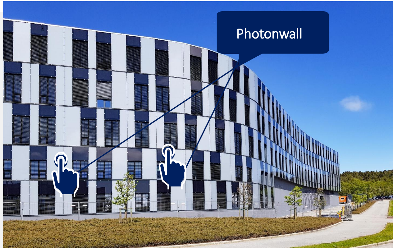
Project for Norwegian Petroleum Directorate Office Building in Stavanger, Norway. Completed in 2019/2020, 1000m 2 ventilated façade PhotonWall. After few years of service it is producing 28% more energy than expected.
