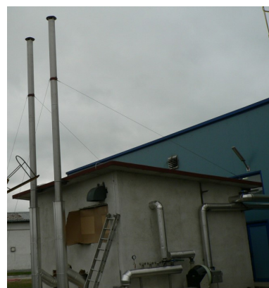
The boiler house with 2 water heating boilers total 550 kWth
