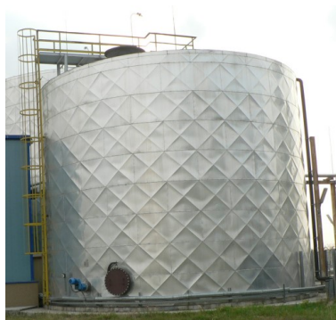
The buffer tank 600 m 3
