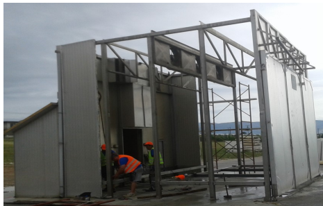
Assembly of 1-st wood kiln dryer
