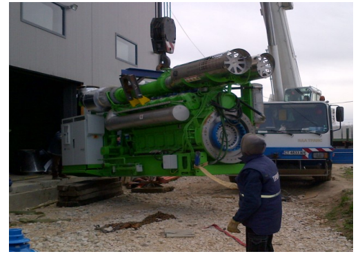
Mounting of cogeneration engines
