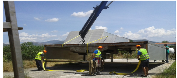
Disassembly of 2-nd wood kiln dryer
