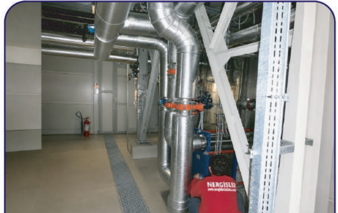
PASLANMAZ SICAK SU HATTI STAINLESS STEEL HOT WATER PIPING LINE
