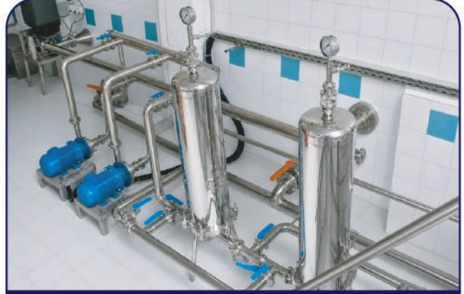
İÇME SUYU FİLTRE GRUBU POTABLE WATER FILTRATION SKID
