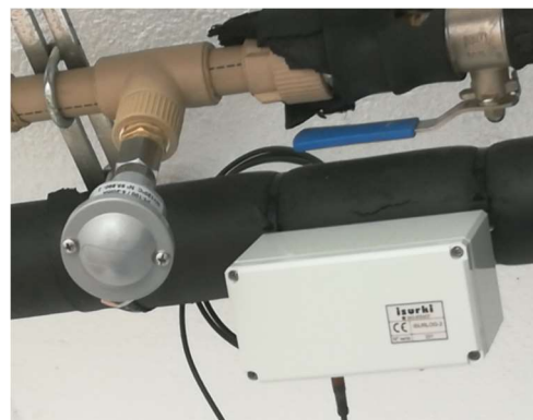
⇐ ↑ ISURLOG NB field unit for HVAC network temperatures monitoring at a health service facility.
