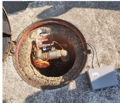
↑ ISURLOG NB field unit for drinkable water distribution network pressure monitoring
