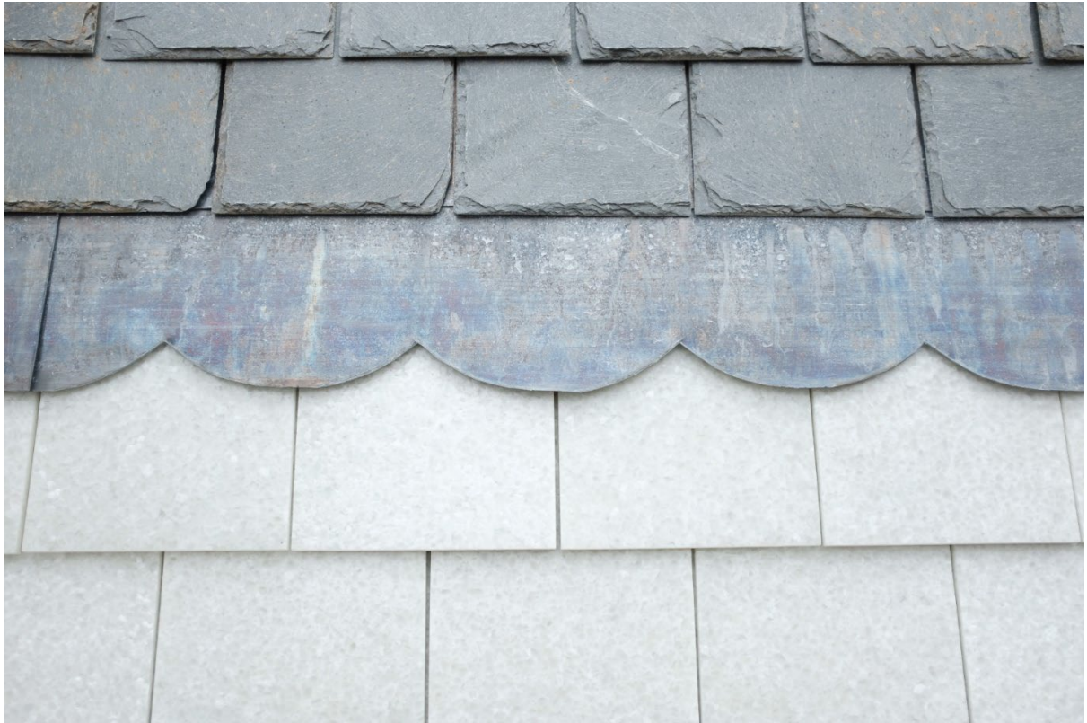
Figure 2, Recycled glass integrates with the traditional slate shingles
