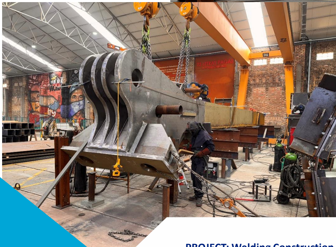
PROJECT: Welding Construction - Colombo Shopping Center (under construction) PLACE: Lisbon, Portugal
