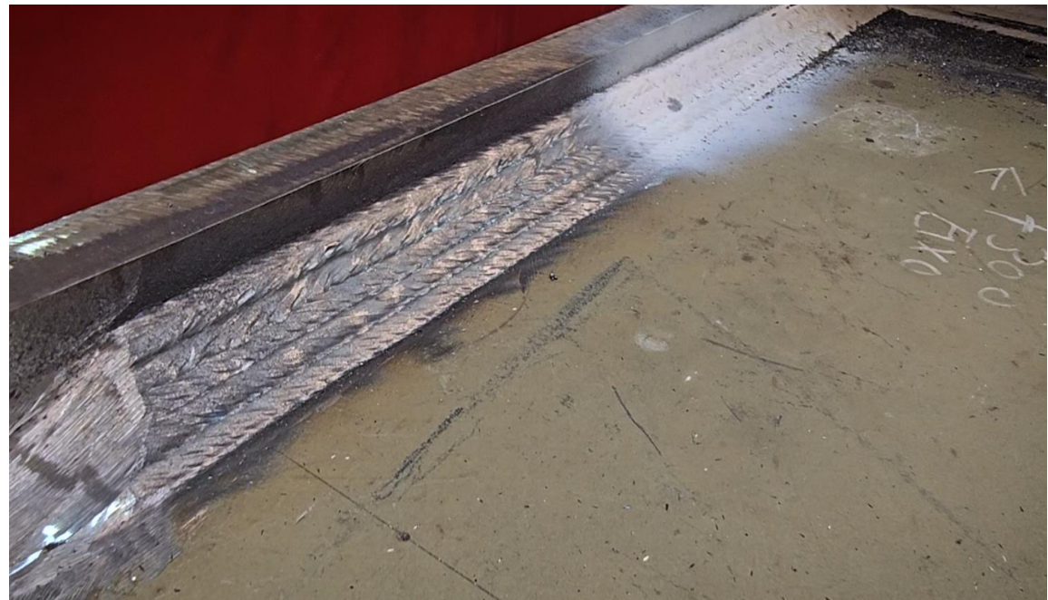
PROJECT: Welding Construction - Colombo Shopping Center (under construction) PLACE: Lisbon, Portugal
