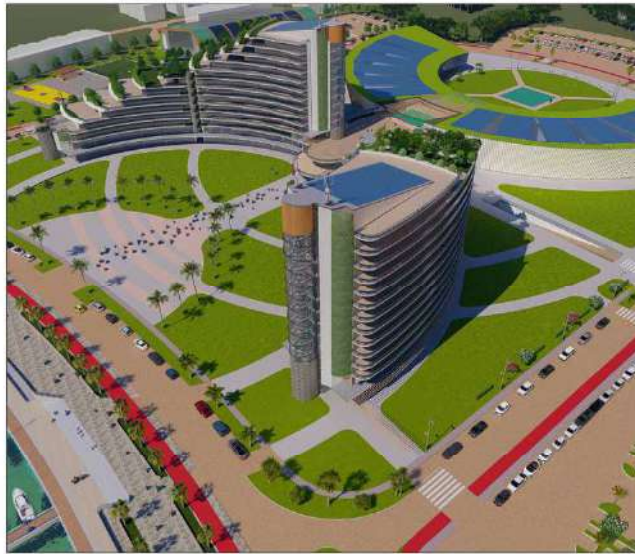
General View of the Residential/Hotel Area
