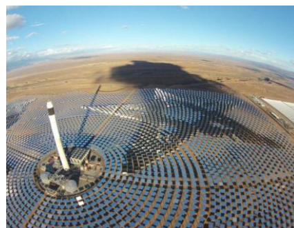
Hybrid complex CSP+PV Noor Middelt 800 MW (Morocco)
