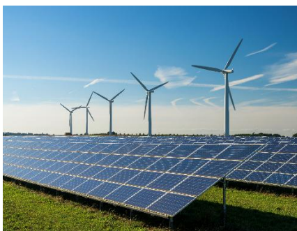
Hybrid complex Wind+PV+Storage Heolios 900 MW (Chile)
