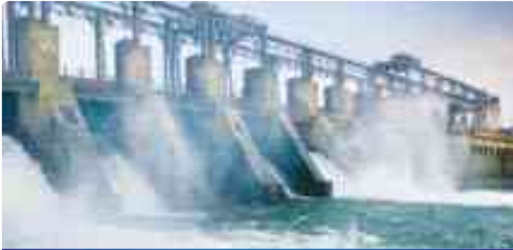
Hidro-Elektrik Enerji Santralleri Hydro-Electrical Power Plants
