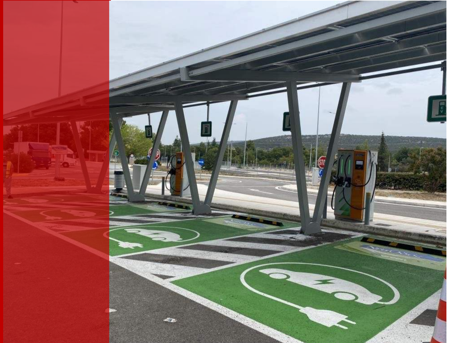
E2C SRL - Conversion system composed by a PV plant with an energy storage system for powering a charging station for EV in the highway.
