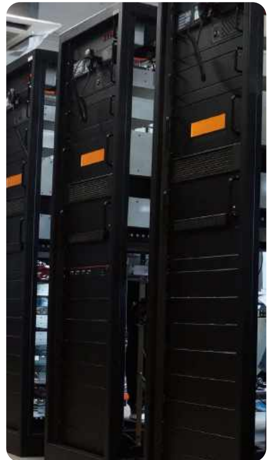
Example of multiple-racks for large scale solutions.
