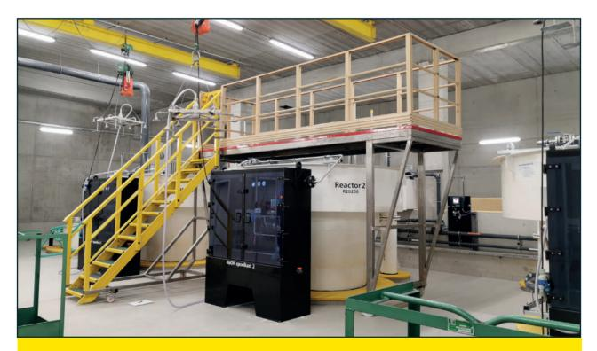
The picture above shows a mobile solution based on three different materials: stainless steel, isophthalic polyester and vinyl ester.
