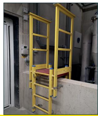
All solutions can be produced using isophthalic polyester resin or vinyl ester resin for highly aggressive environments.
