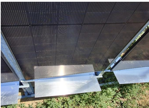
Fig 5: Reflective gutter
