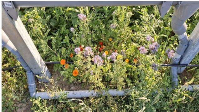
Fig 7: Protective plants under the solar panels
