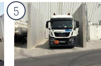
Hydrogen filling station
