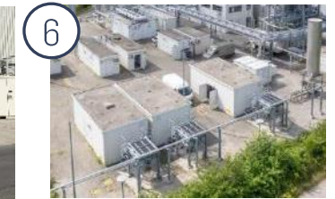
Grid injection plant
