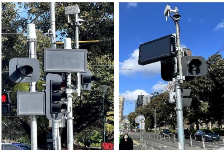
Figure 2: Kapsch RSU and CCTV Installation (Source: Kapsch TrafficCom)
