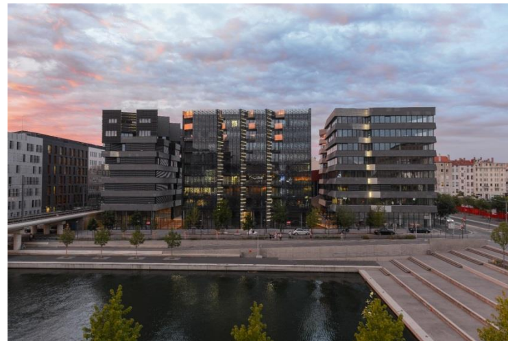
HIKARI - 12 000 m 2 zero energy building in the Lyon-Confluence area in Lyon Photography not to be used without prior authorisation
