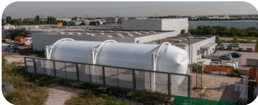
Demonstration plant in Austria (2016)
