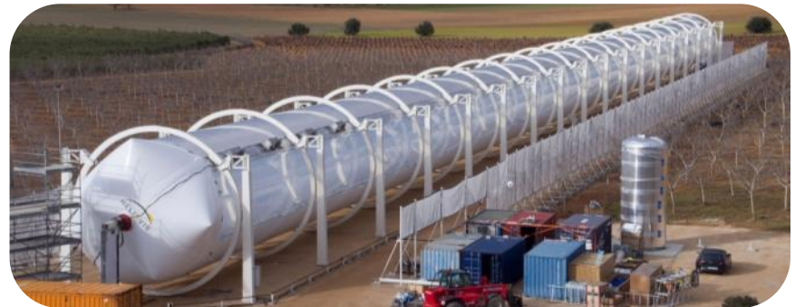
Industrial application in Spain (2016)
