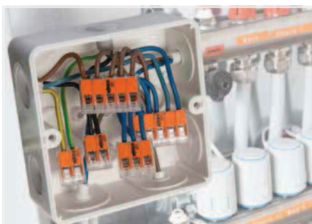
Wiring fine-stranded conductors in a junction box.
