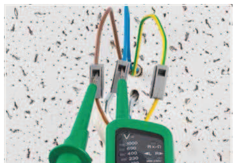
Testing via separate test ports.
