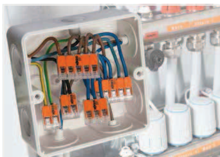
Wiring fine-stranded conductors in a junction box.
