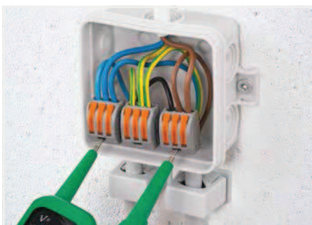
Testing the wired connectors
