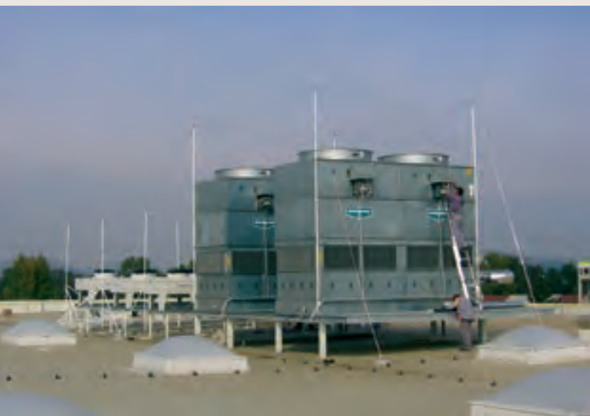
Fixing insulated supporting elements to electrical devices
