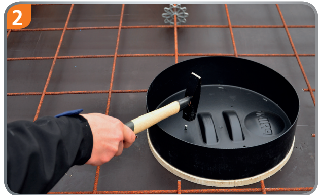
Nail the light-box cover on the formwork.
