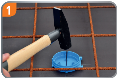
1 Nail the cover on the formwork.
