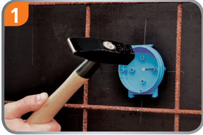
1 Nail the cover on the formwork.
